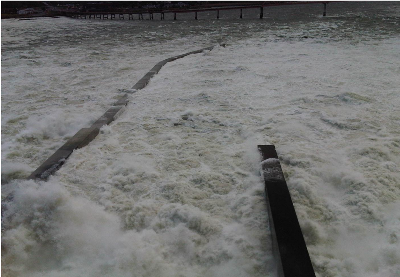
Did we mention high river flow? Over 200 KCFS spill. Spillwall is still standing. High recirculation flow south of wall.
